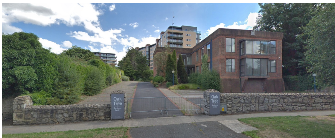
Figure 2.3 - View of Oaktree Business Centre - to be demolished
